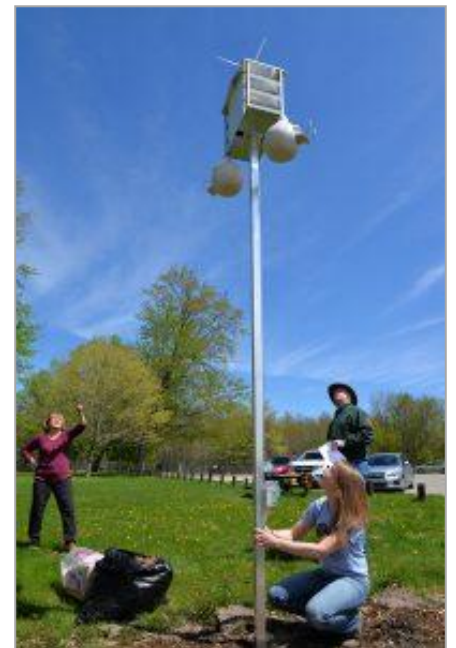
Michigan Audubon Conservation Science Coordinator Rachelle Roake works with dedicated volunteers Rick and Penny Briscoe to install a Purple Martin house at the Ingham County Parks Lake Lansing boat launch.
